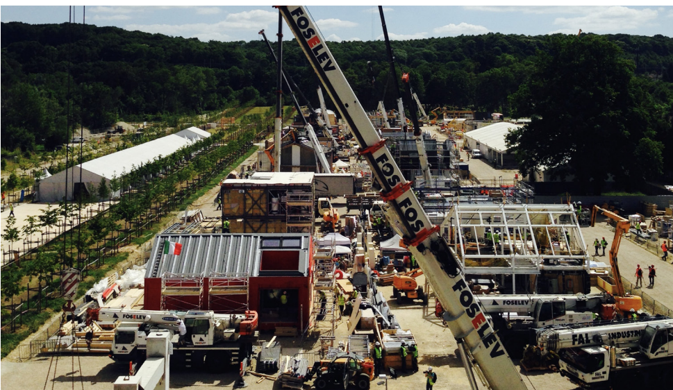
SDE14 CONSTRUCTION PHASE © VALERIA ANZOLIN, SDE14
